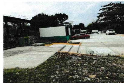
F3: Barda perimetral
