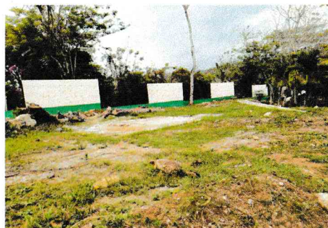
F4: Barda perimetral
