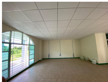
F2: Interior aula
