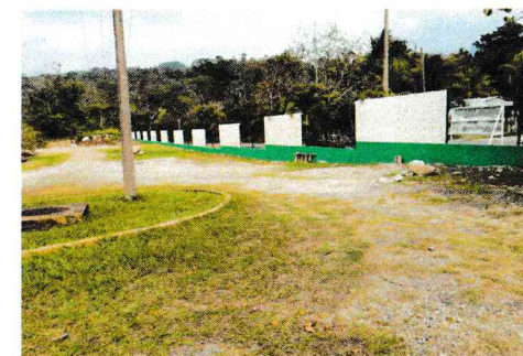
F5: Barda perimetral
